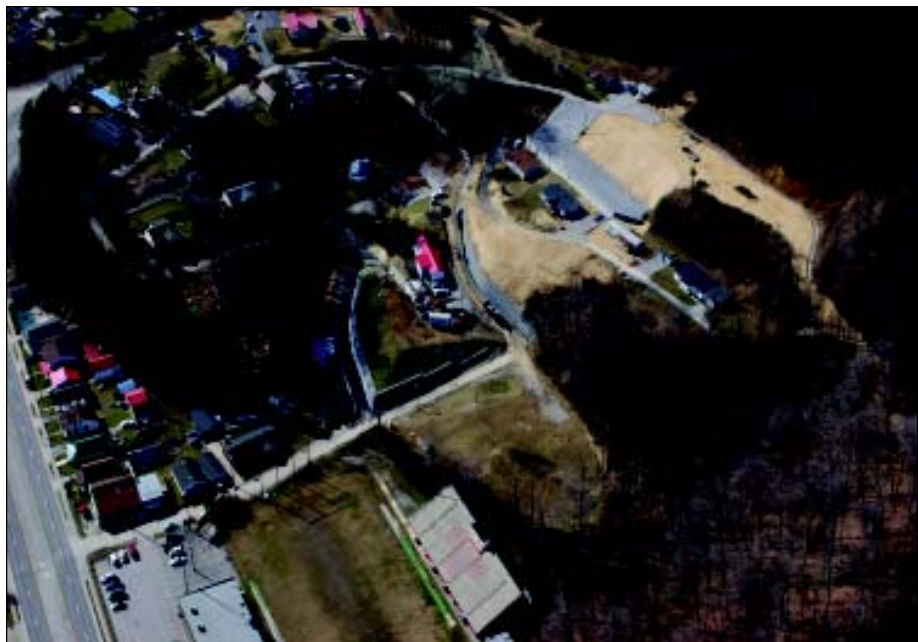
The AML built retaining walls (upper right) to protect surrounding homes and the Belfry High School (lower left) from a landslide. AML photo
